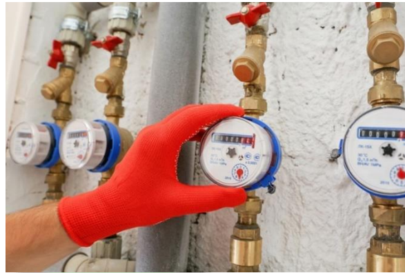
Gambar 3. 10 Water sub metering Sumber : (verdriver.org, 2022)
