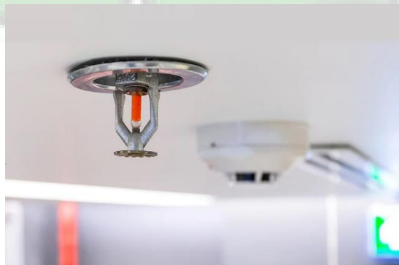
Gambar 5. 28 Sprinkler (Sumber: sfpe-qatar.org)
