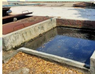
Gambar 2.2 Sumur Endapan Air limbah RPH
