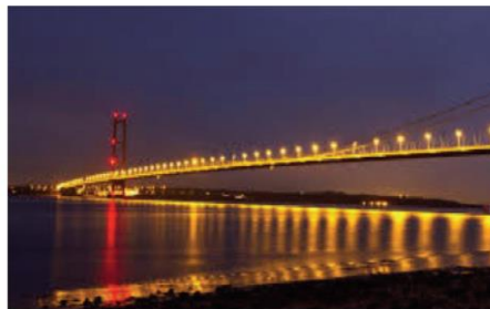
Source: www.nelpis.wordpress.com Picture 11.1 Humber Bridge
